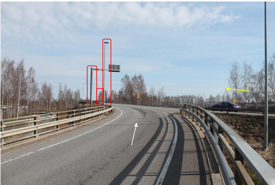
Pos 7/Pic 30. Turning from road 2 toward road 8. Marked lamp posts and portal need to be removed. Marked trees need to cut. Rails height 1,06m. Blade need to be lifted and need to be able to oversail the rails. White arrow points driving direction for blades on counter lane. Yellow arrow points driving direction for towers etc.
