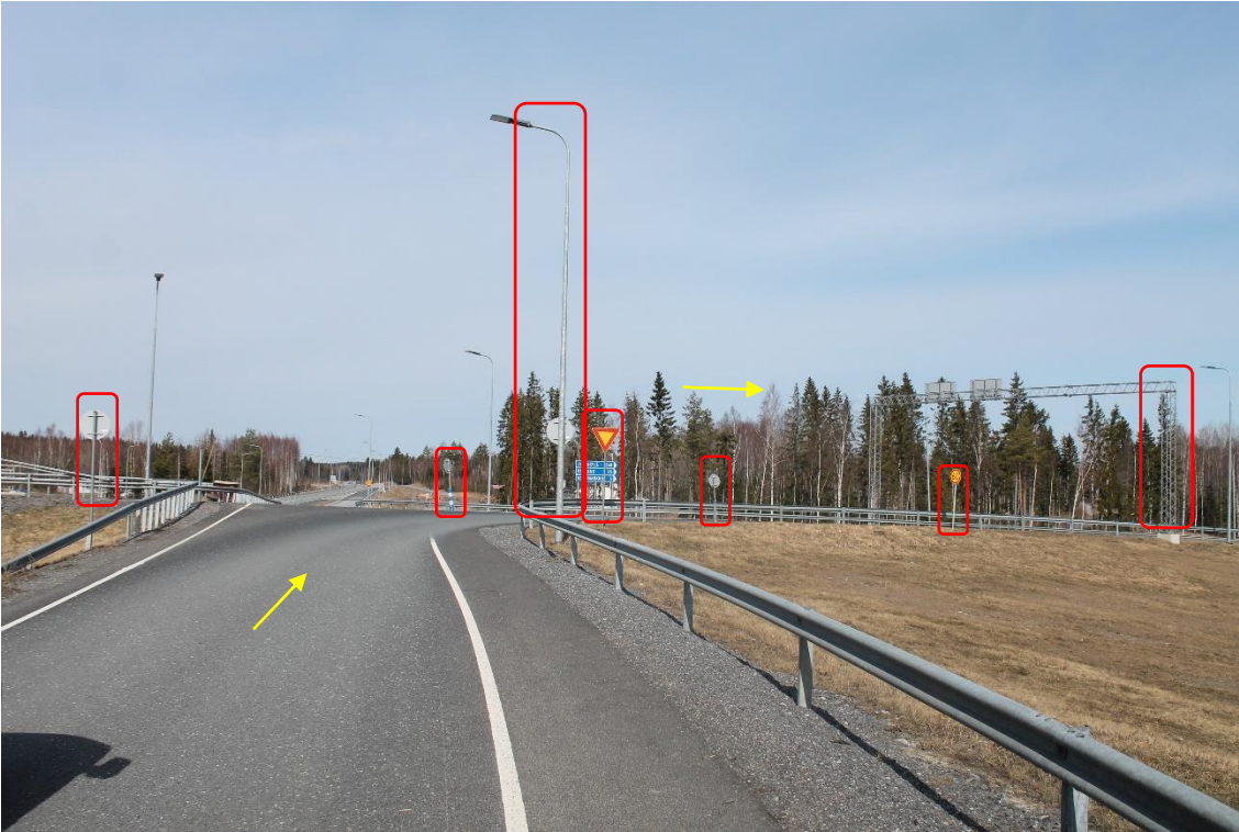
Pos 10/Pic 37. Turning from road 8 toward road 23. Marked lamp post, portal and signs need to be removed. Rails height 0,7m.
