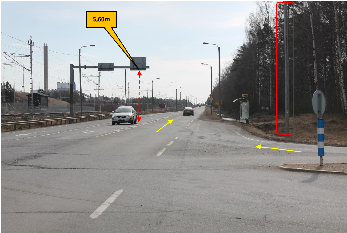
Pos 3/Pic 11. Road 2. Bridge detour on road 2. Marked Lamp post need to be removed.
