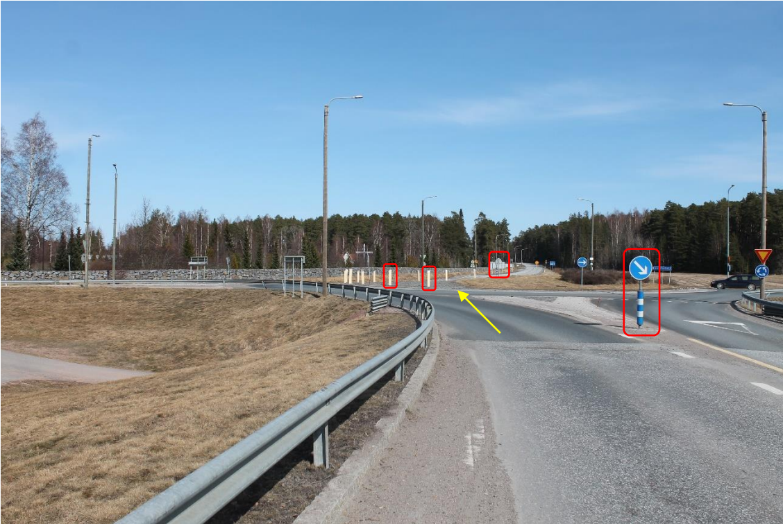
Pos 12/Pic 43. Road 23 roundabout in Noormarkku. Need to drive thru on counter side. Marked signs and poles need to be removed.
