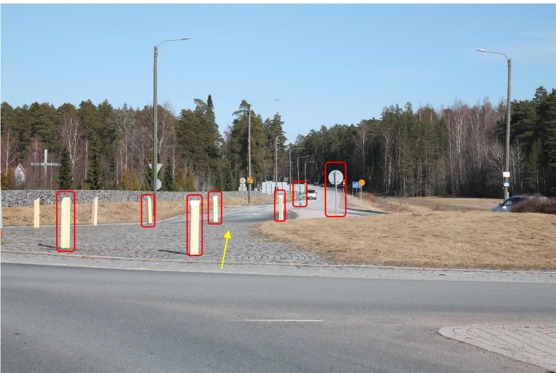
Pos 12/Pic 44. Road 23 roundabout in Noormarkku. Need to drive thru on counter side. Marked signs and poles need to be removed.
