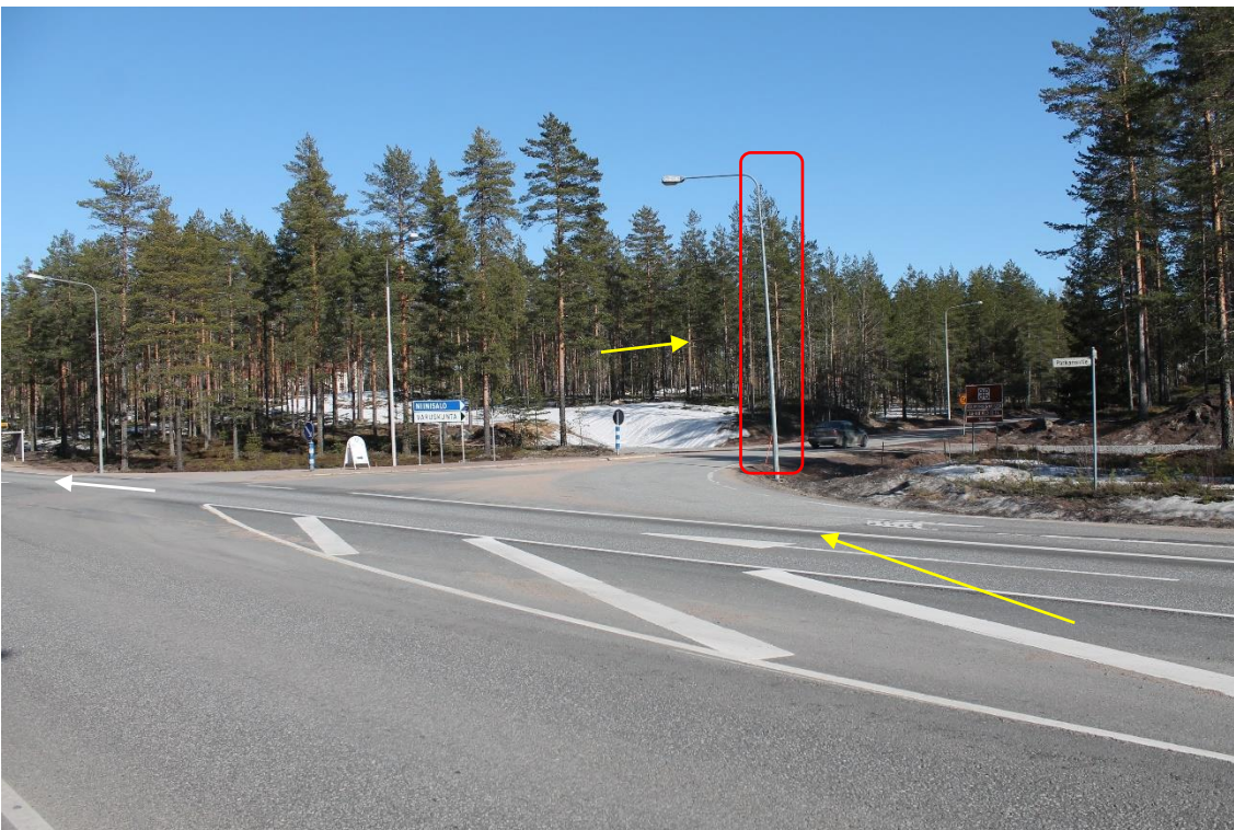
Pos 15/Pic 50. Turning from road 23 toward Varuskunnantie. Bridge detour. Marked lamp post need to be removed. White arrow points driving direction for blades. Yellow arrow points driving direction for towers.
