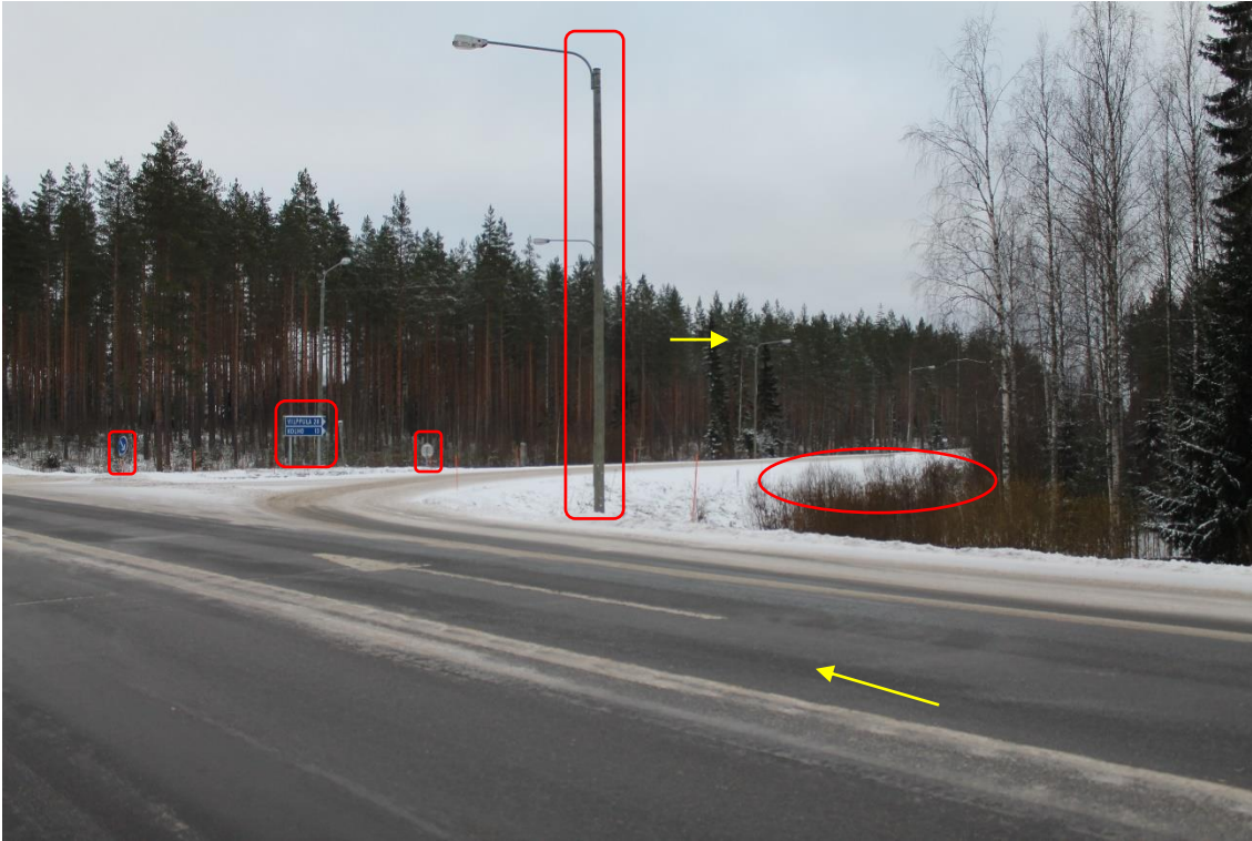
Pos 36/Pic 91. Turning from road 23 toward road 3482. Marked signs and lamp posts need to be removed. Marked bushes need to cut.
