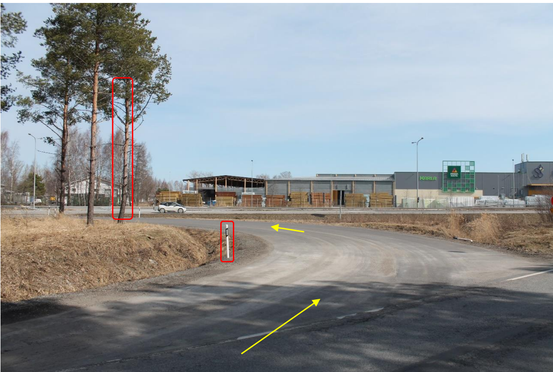
Pos 7/Pic 20. Turning from road 2 toward road 8. Transports need to make u-turn on designed ramp to road 8. Marked tree need to cut. Marked pole need to be removed. Yellow arrow points driving direction for towers etc.
