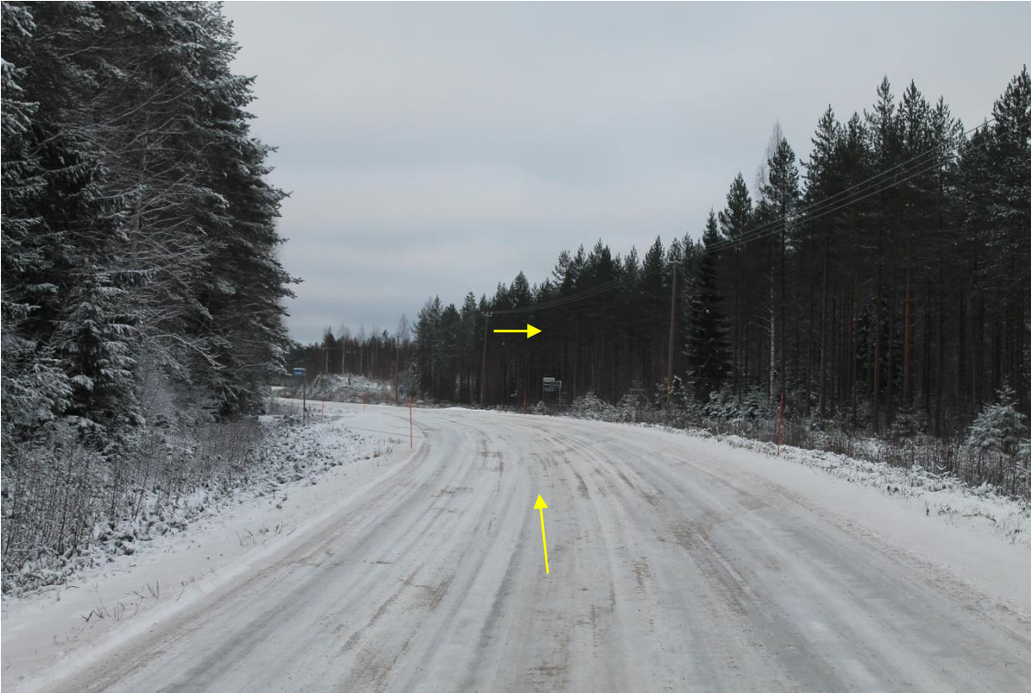
Pos 38/Pic 93. Turning from road 3482 toward Ristimäentie. https://maps.app.goo.gl/ztSVwHy169P35UAS6 This junction to be considered as new site entrance. Site entrance to be build according to specifications for site roads. Original site entrance is not feasible.
