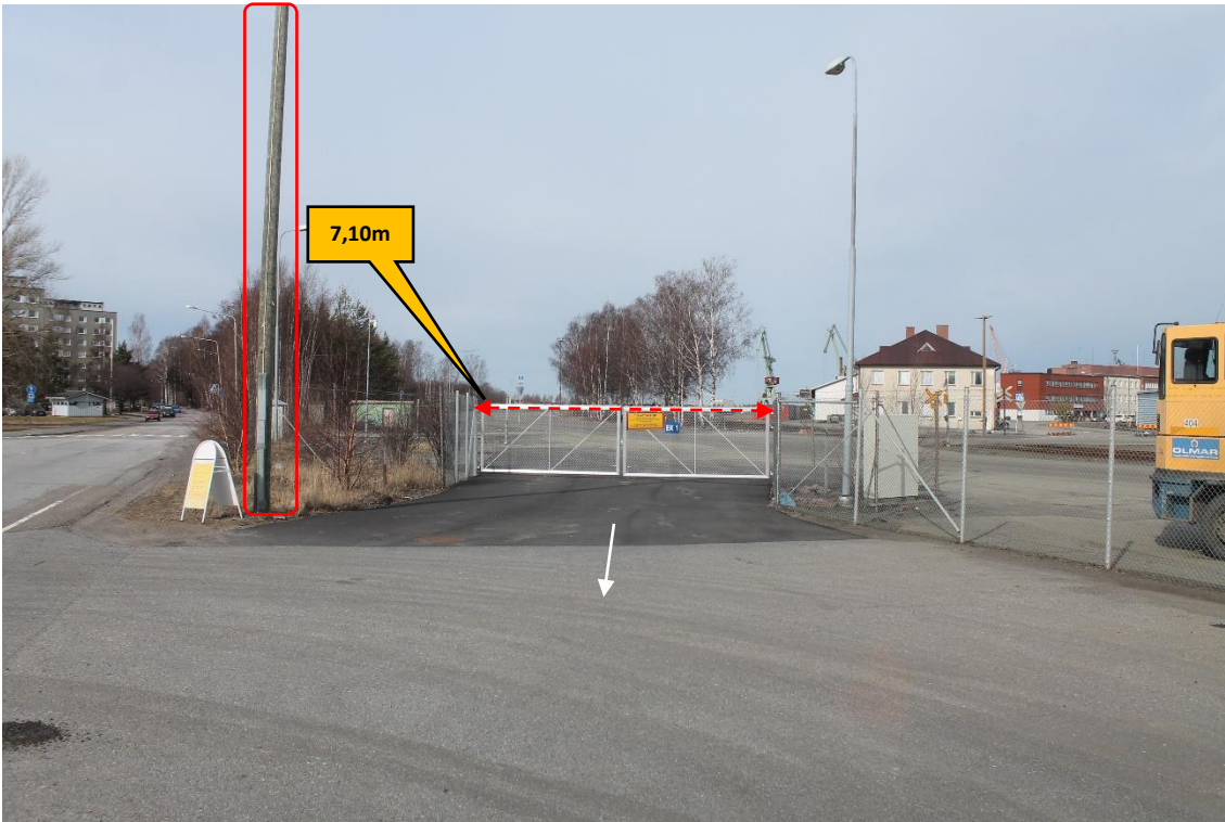
Pos 1/Pic 1. Exit from port via gate EK1. https://goo.gl/maps/BamiPLb9PiQk4WWk7 This gate to be used for blades. Marked lamp post need to be removed.
