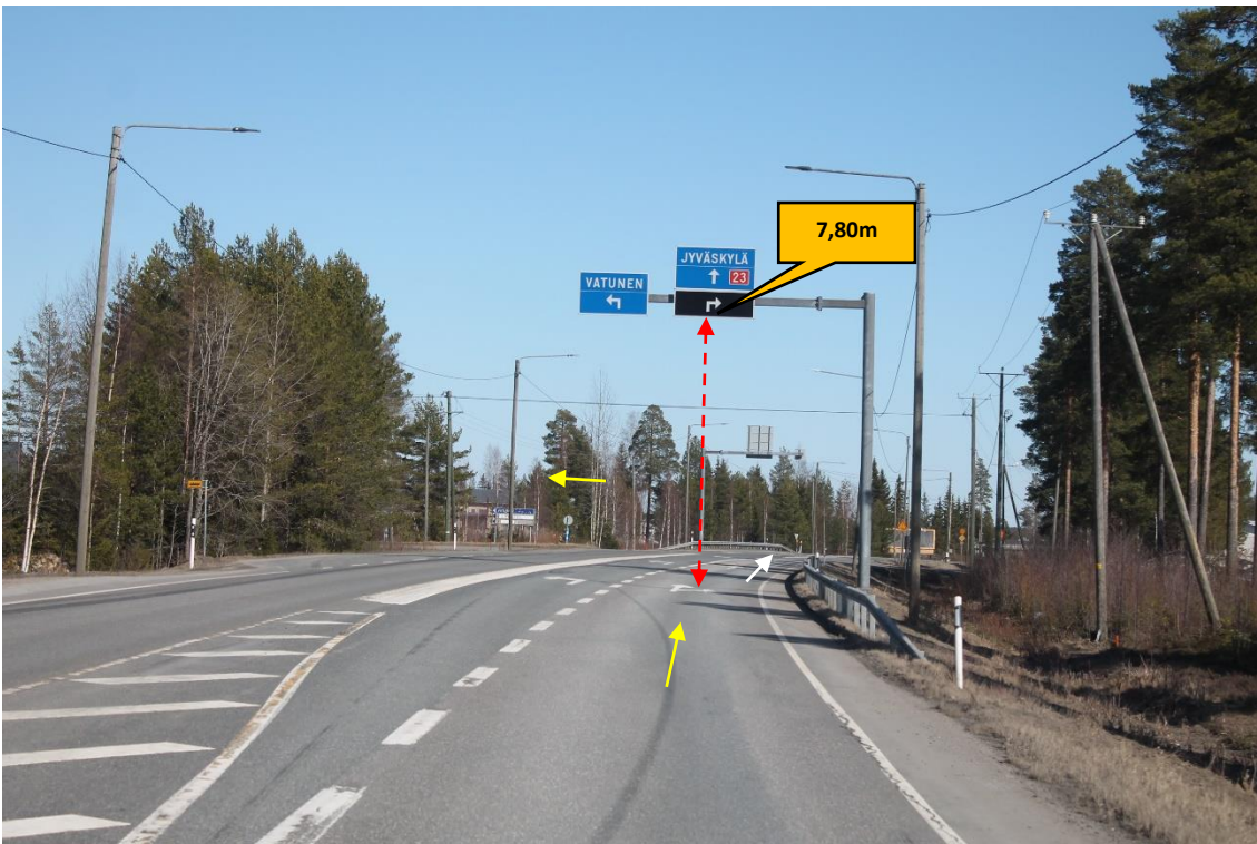
Pos 23/Pic 64. Road 23. https://goo.gl/maps/fCDyKbaw3zcksk2X7 Yellow arrow points driving direction for towers. White arrow points driving direction for blades.
