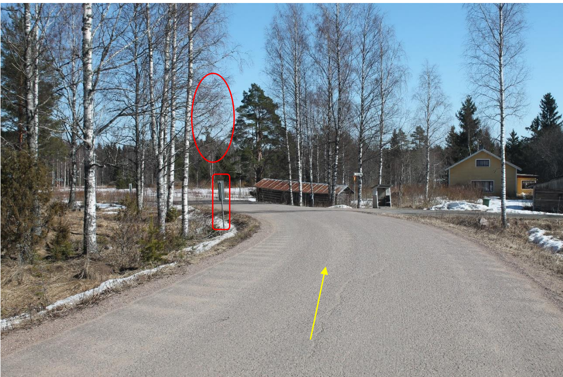
Pos 21/Pic 60. Rautalammentie. Bridge detour. Marked sign need to be removed. Marked tree branches need to cut. Yellow arrow points driving direction for towers.
