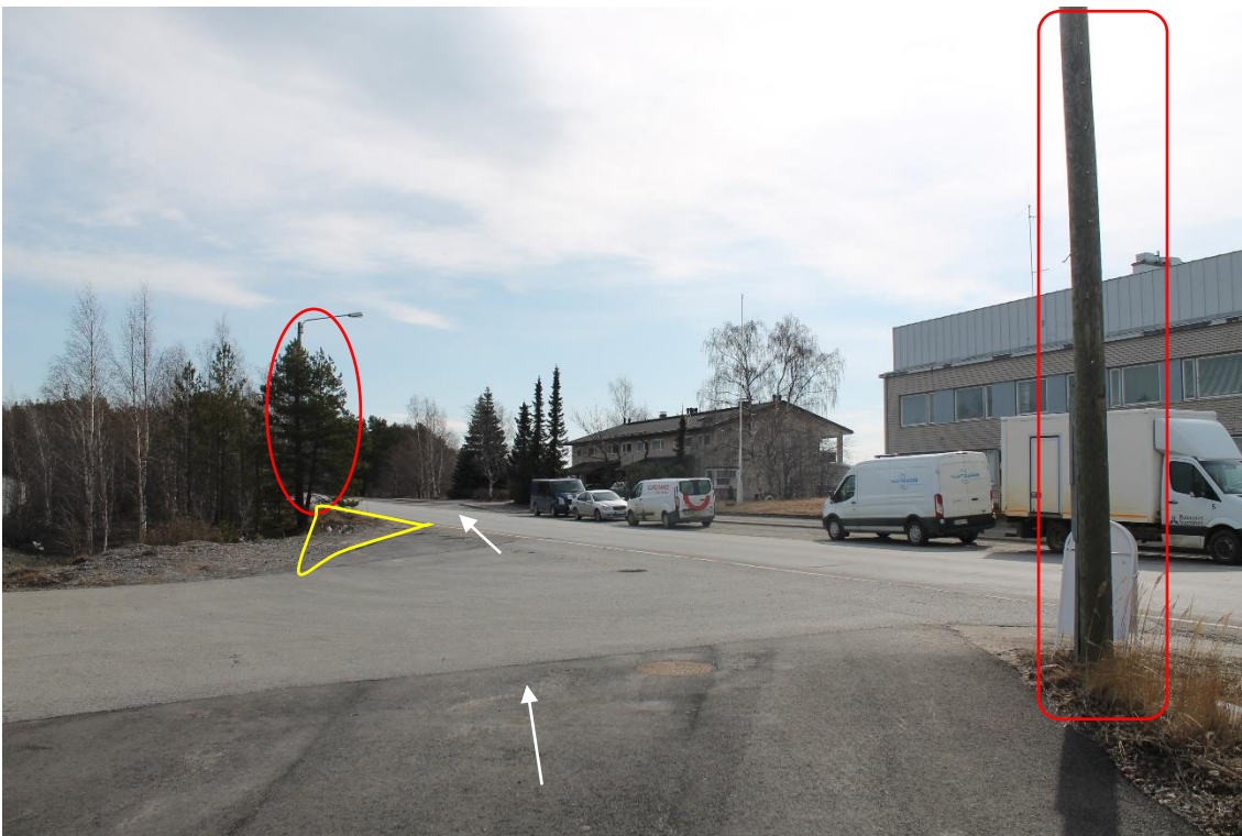
Pos 1/Pic 2. Exit from port via gate EK1. Marked trees need to cut. Marked lamp posts need to be removed. Marked area need to be filled and drivable.
