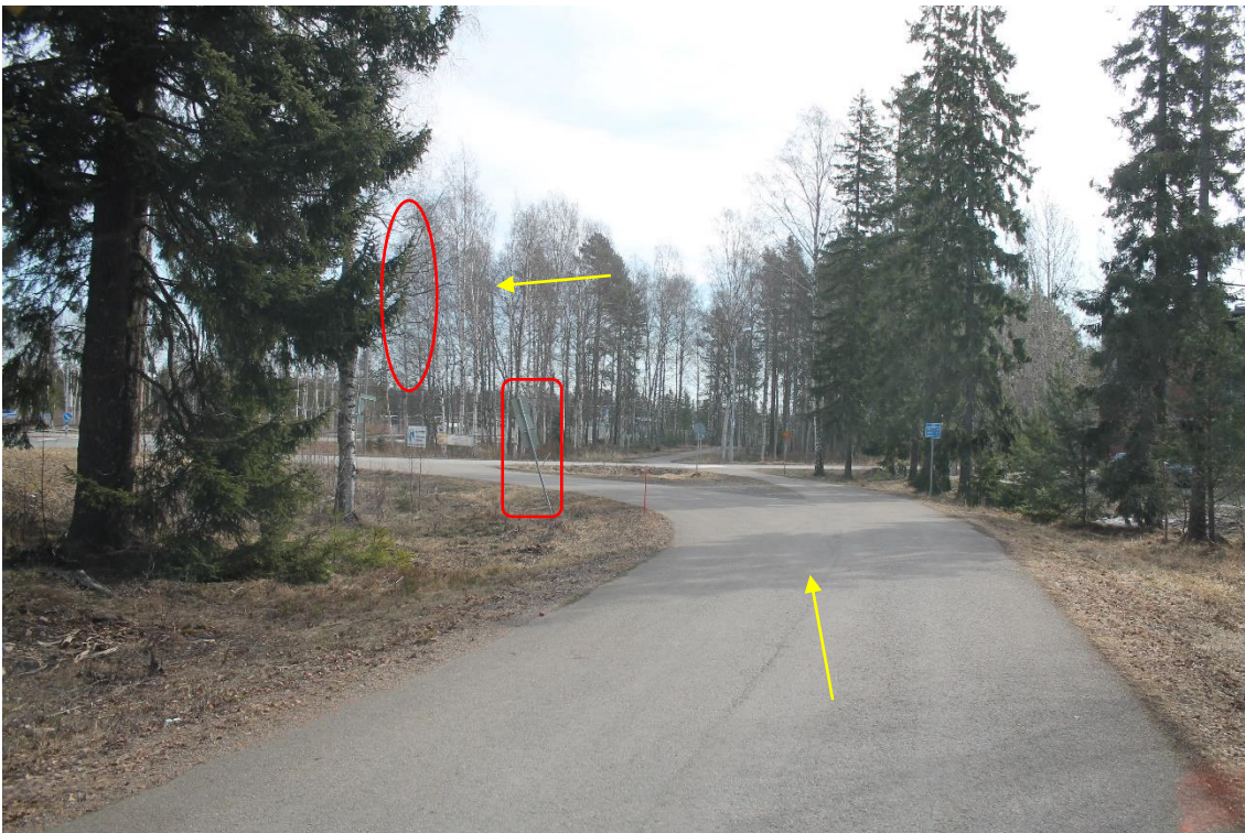
Pos 3/Pic 8. Bridge detour on road 2. Marked sign to be removed. Marked tree branches need to cut.
