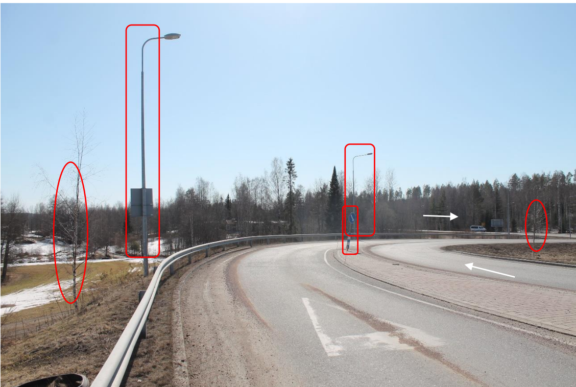
Pos 25/Pic 70. Turning from road 23 toward road 3. Marked signs and lamp posts need to be removed. Marked trees need to cut.
