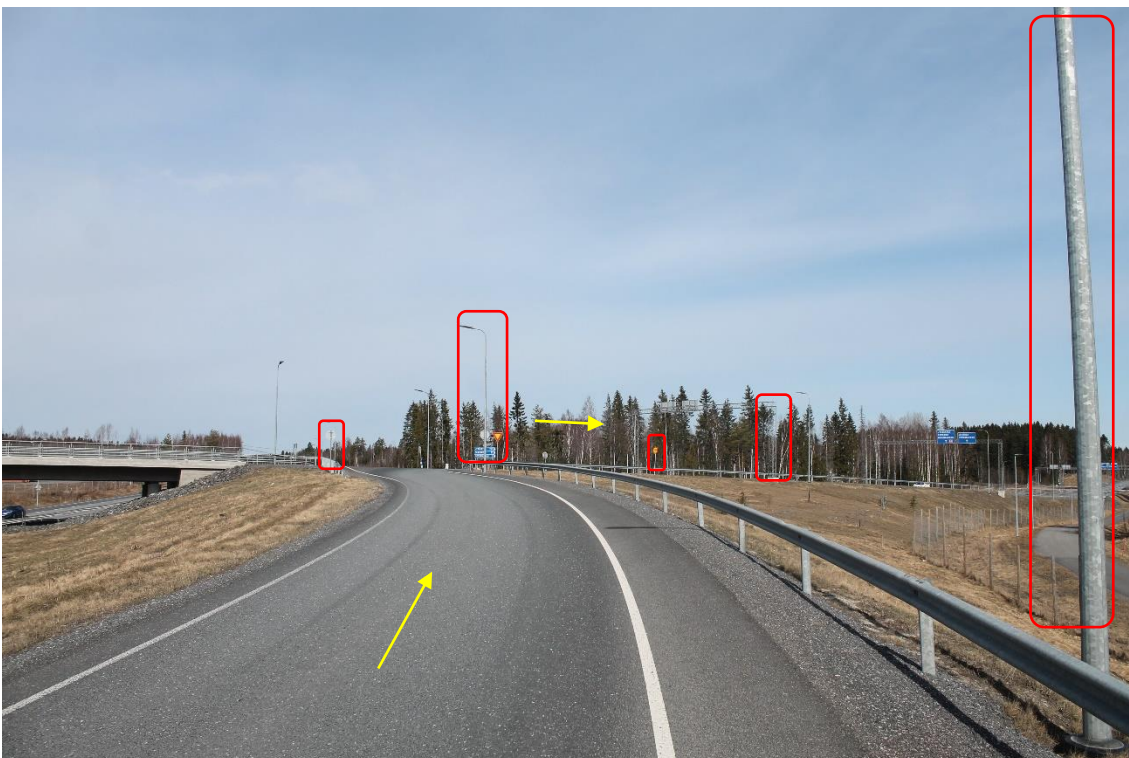
Pos 10/Pic 36. Turning from road 8 toward road 23. Marked lamp posts, portal and signs need to be removed.
