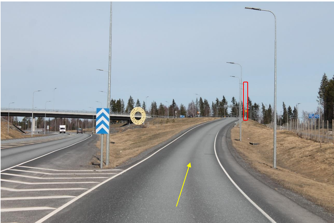
Pos10 /Pic 34. Turning from road 8 toward road 23. https://goo.gl/maps/AxWKWiPAL1THNcKP8 Marked lamp post need to be removed.
