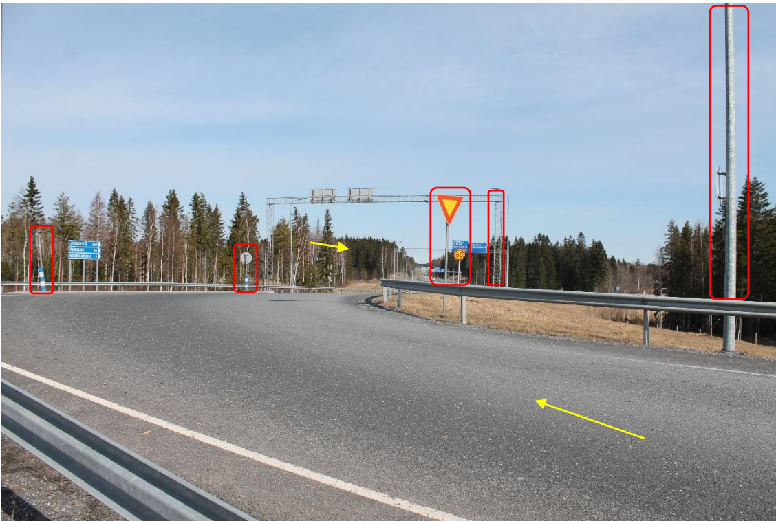
Pos 10/Pic 38. Turning from road 8 toward road 23. Marked lamp post, portal and signs need to be removed. Rails height 0,7m.
